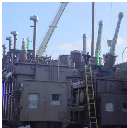
Phase angle regulator | Con Ed
