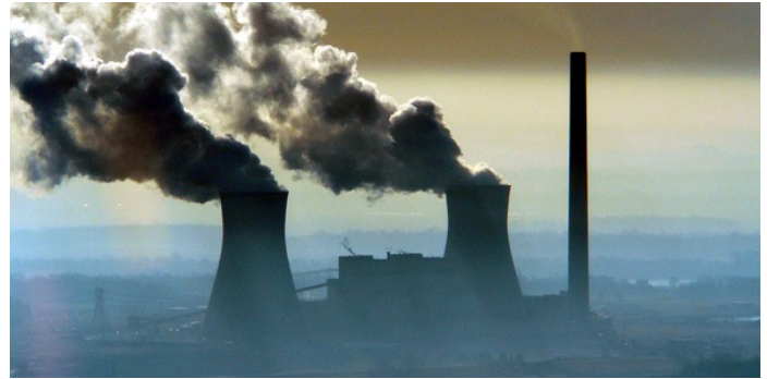
Rockport Generating Station | © John Blair
